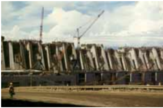
The construction of Itaipu 1981
